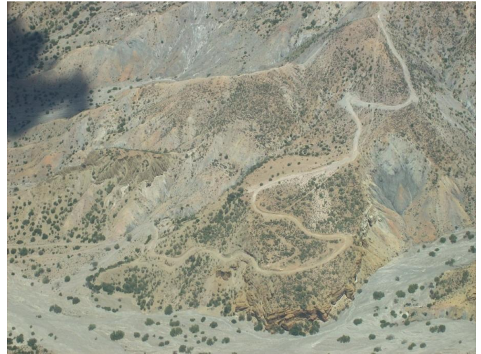
Completed Road: Sagrario to Cayti
