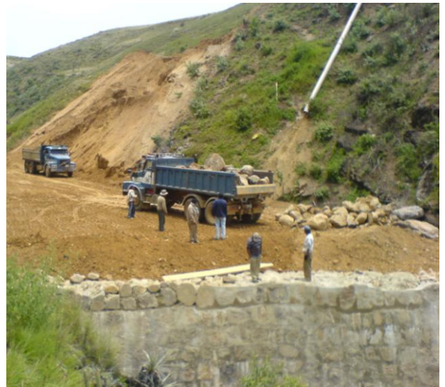
Building lower portion of reservoir retaining wall
